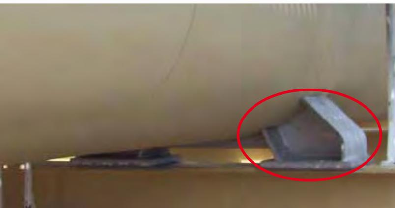
3. ALL STEEL WORK CONNECTED DIRECTLY TO THE MAIN INSTALLATION MUST BE INSULATED TO THE SAME THICKNESS AND COMBINATION OF INSULATION MATERIALS SO AS TO AVOID ACOUSTIC BRIDGING AND MAINTAIN OPTIMUM PERFORMANCE.
